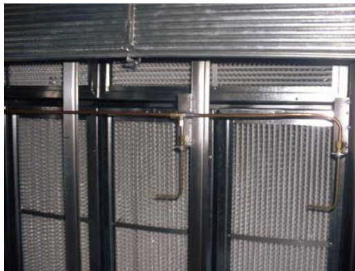
Pressure Transmitter Locations Figure 6
